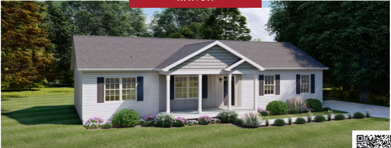
Shown with site built porch.
